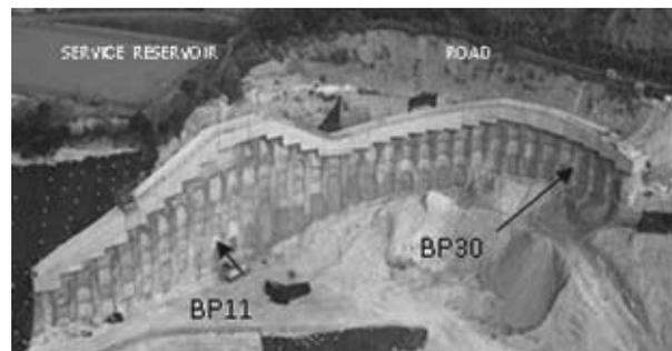
Figure 4 Bored-pile wall in Hong Kong (after Ho et al. 2013).
