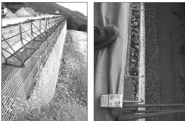
Figure 8. Left: construction stages (formwork, geogrids, anchor bars, facing), right: top view of the stone-filled facing used.
