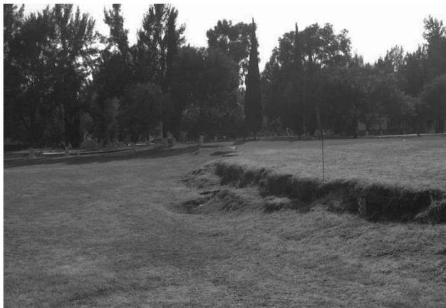
Figure 7. Crack in an abrupt transition area.
