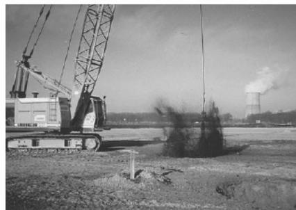
Figure 2. Compaction of deposited waste by dynamic consolidation
