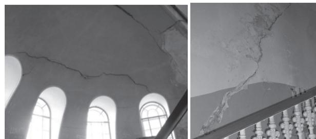
Fig. 6. Cracks in the vaults of the cathedral
