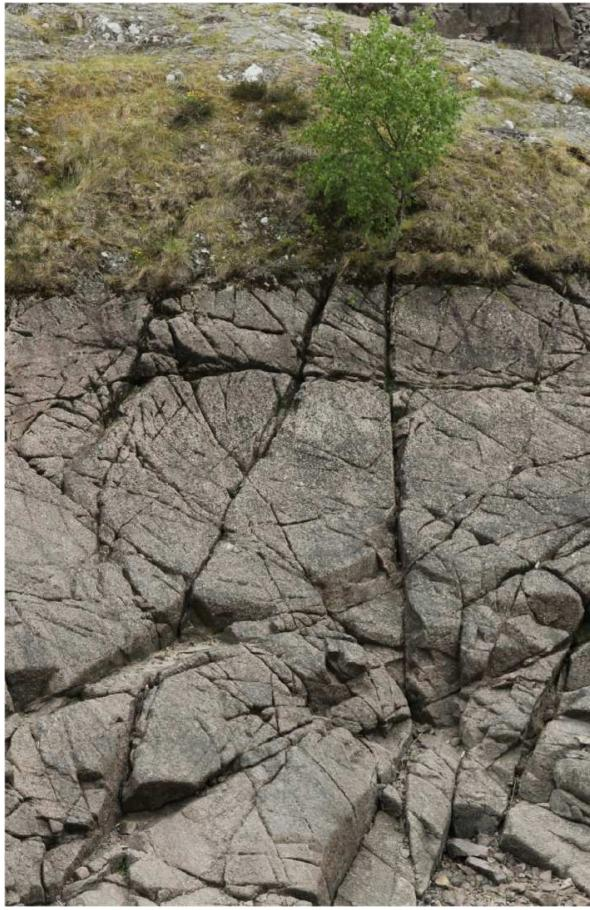
Figure 2. A typical view of superficial fracturing in a microgranite. Taken at the Alfeld Dam right bank abutment in Upper Rhine District, France.
