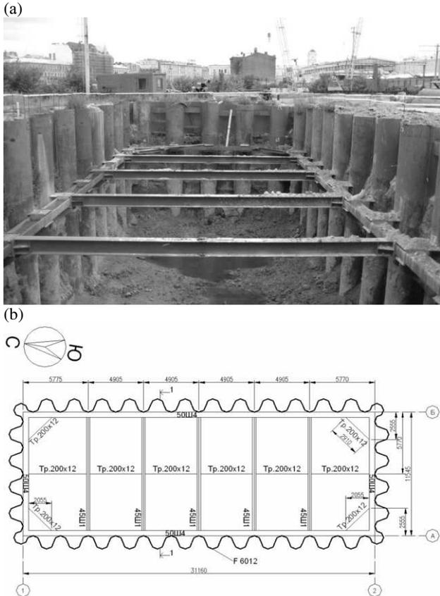
Figure 2. Overview (a) and (b) layout of sheet piles and beams at the level of -3.5 m from the sheet piles top at the test pit.
