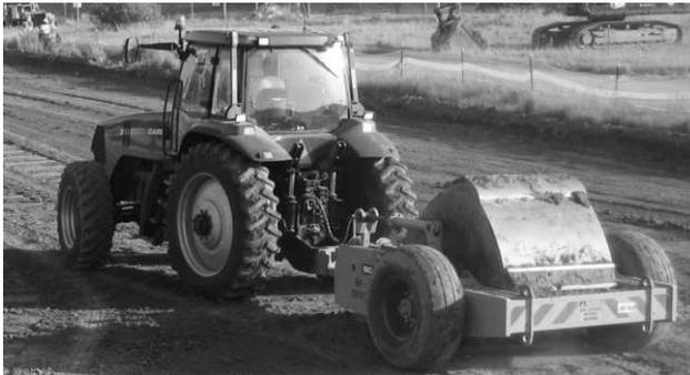
Figure 2. Impact rolling in progress.
