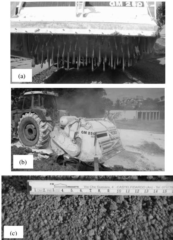
Figure 4. Soil-lime mixture test pad: tilling equipment (a), spreading of lime on the surface of a 35-40 cm thick lift and first mixing (b), soil-lime mixture after 3 passes of tiller.
