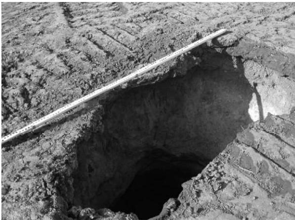
Figure 1: Sinkhole during construction.
