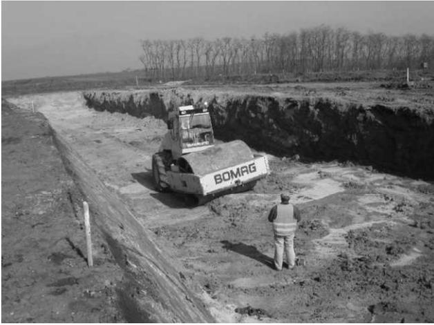
Figure 10: Remote-controlled Vibration Roller
