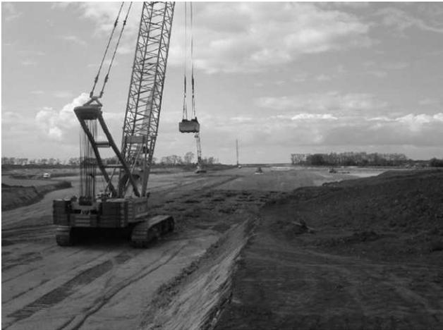
Figure 11: Dynamic Compaction Works
