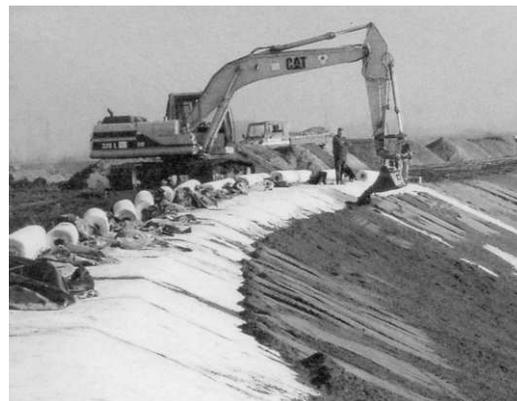
Figure 3. Lippe River dike rehabilitation (1994): installation of Bentofix GCL as a sealing layer
