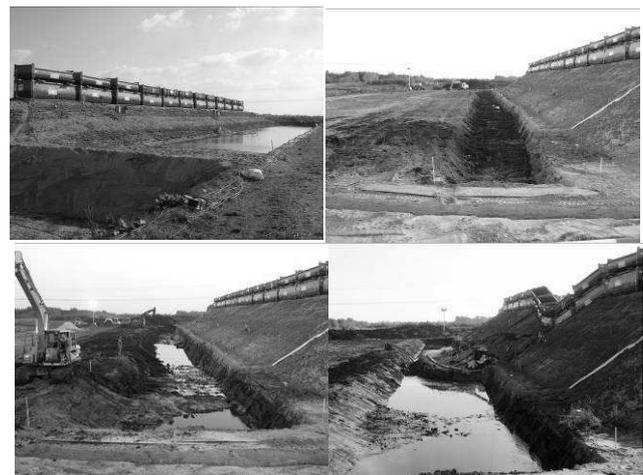
Figure 17 a) River side of the dike, b) Inner side of the dike during excavation of the ditch, c) Inner side of the dike after excavation of the ditch, d) Failure
