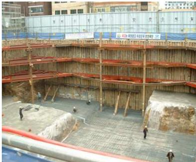
Photo 2. IPS earth retention system in urban excavation
