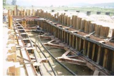
Photo 1. IPS earth retention system in trench excavation
