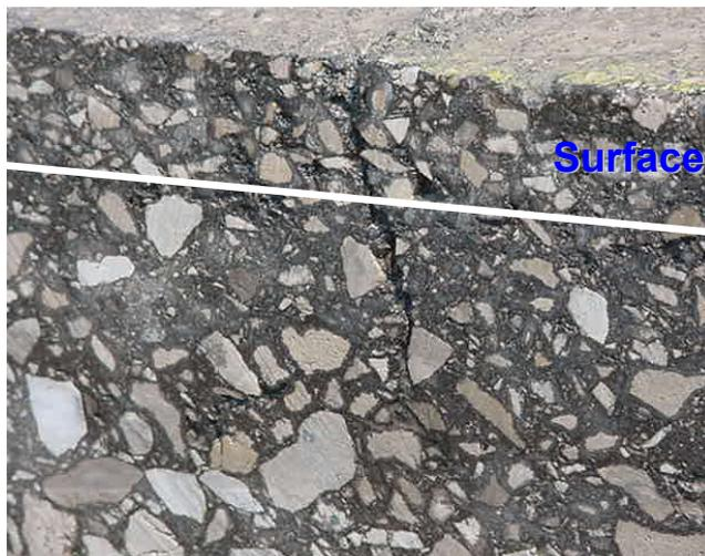
Figure 2. Top-down longitudinal crack and segregation of surface layer
