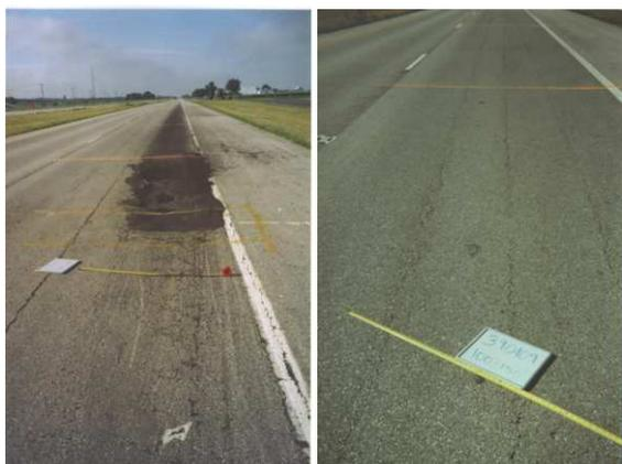
Figure 1. Distress photograph of Section 390103 (left) and typical longitudinal cracks (right)
