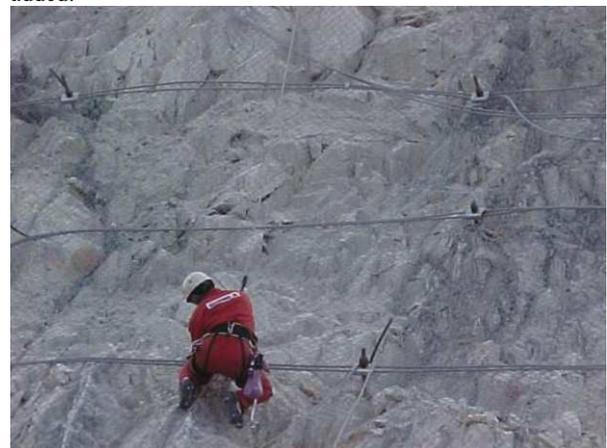
Figure 4. Tecco mesh reinforced by cables (courtesy of Geobruigg)
