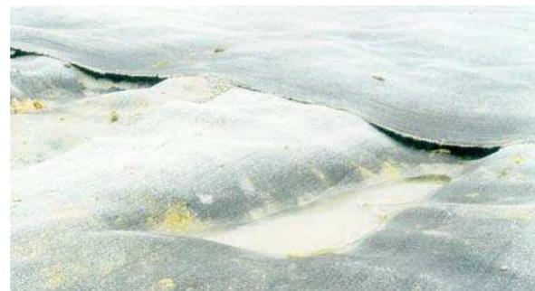
Fig. 5 GCL installed on an irregular/rutted (poor) foundation and not covered before heavy rainfall
