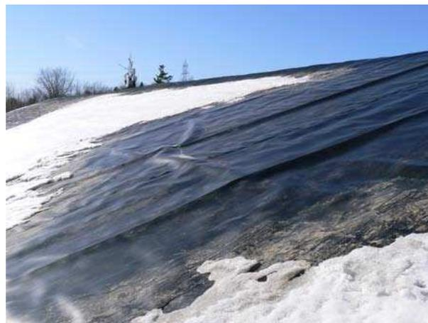
Fig. 8 Geomembrane partially covered by snow but with significant wrinkles in snow free areas on south facing slope
