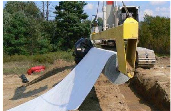
Fig. 2 GCL being unrolled on site as it is installed
