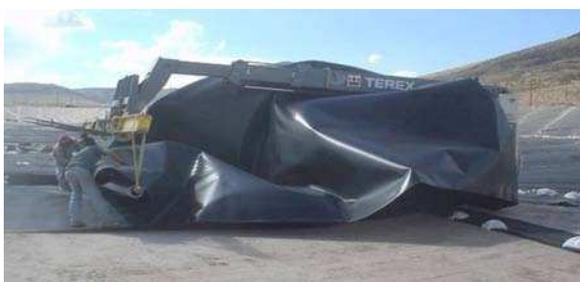
Fig. 7 Geomembrane panel picked up by wind (Photo: courtesy of R. Thiel)
