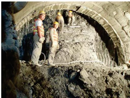
Figure 4. Upper half-section excavation with central part of the face left in place (Tangier face, around PK 27+960).
