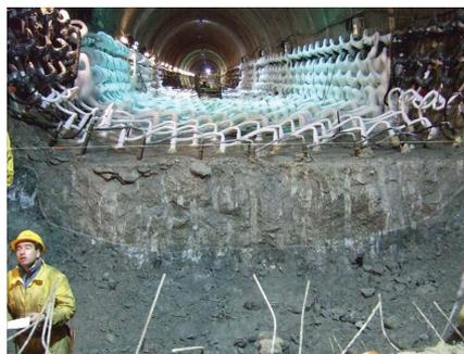
Figure 5. The excavation of the existing invert.
