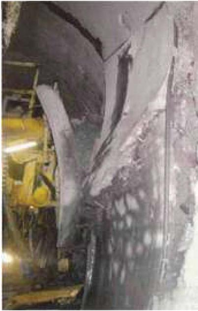
Figure 5. Failure in the Aicha Tunnel, breakage of the left-hand shotcrete lining.
