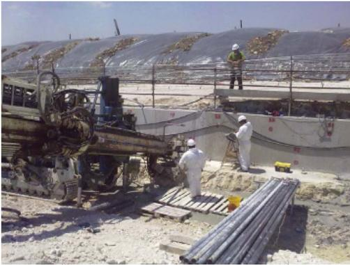
Figure 10. Rigs drilling for grouting.
