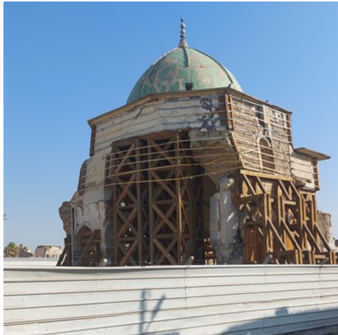
Figure 5. Dome of the Al-Nuri Mosque under rehabilitation
