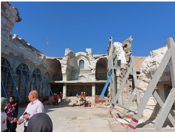
Figure 1. Al-Tahira Church during rehabilitation by UNESCO
