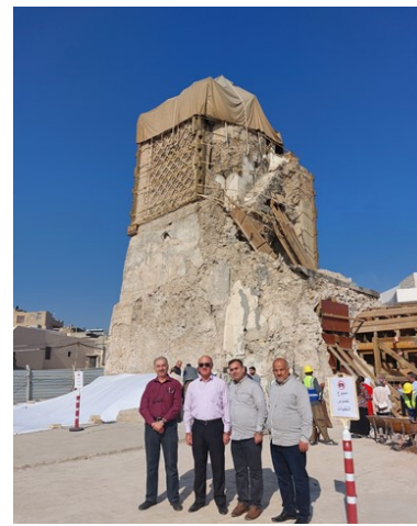
Figure 4. Current view of Al-Hadba Minaret after been destroyed by ISIS
