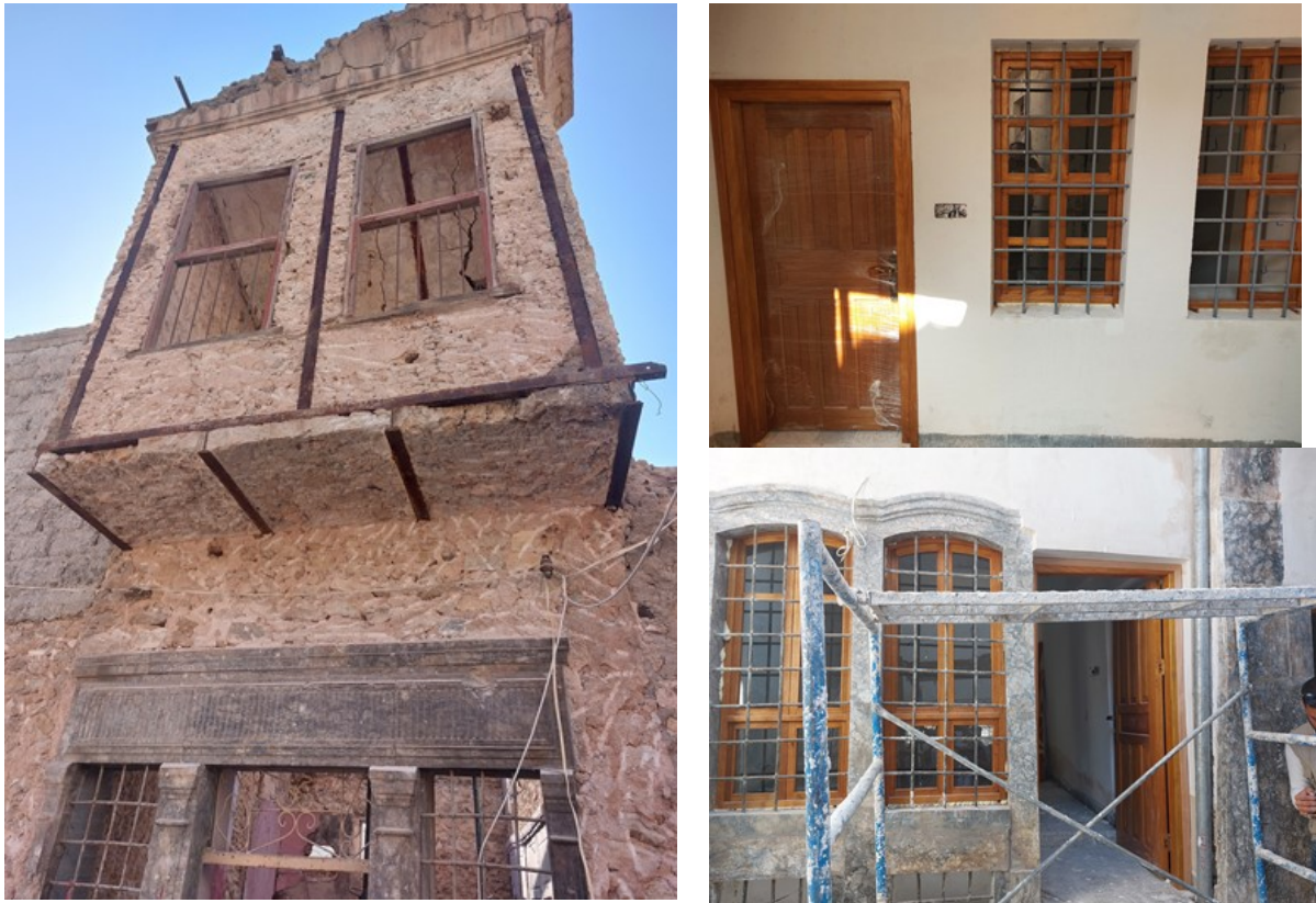
Figure 7. Rehabilitation of one of the historical houses in Mosul old city
