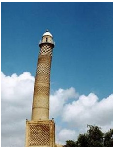
Figure 3. Al-Hadba Minaret inclined with 142 cm from the centerline
