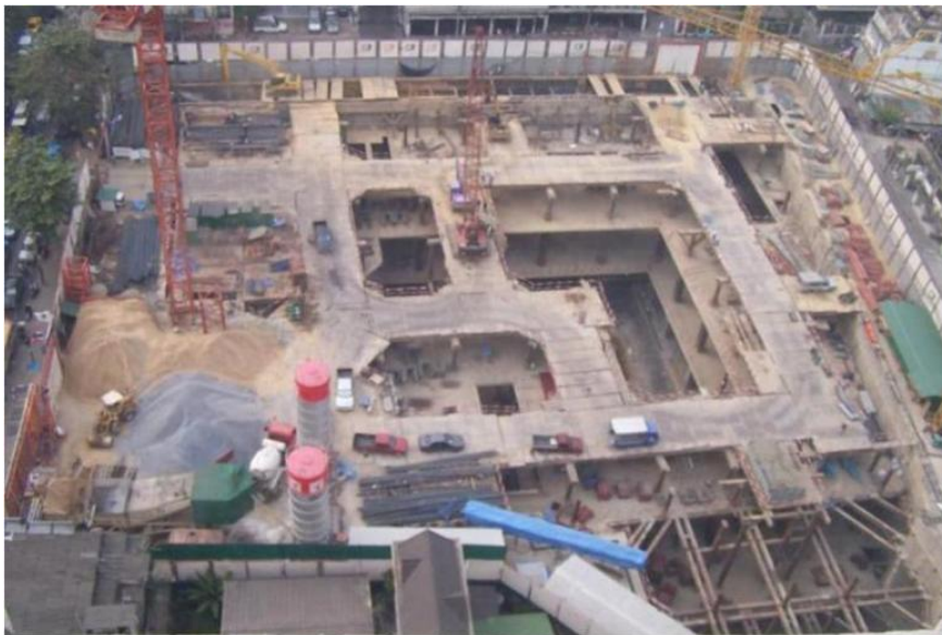
Fig. 2 A boom in utilization of underground space in Bangkok
