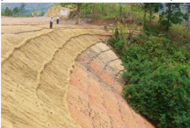
To test the effectiveness of the soil blankets and cushions
