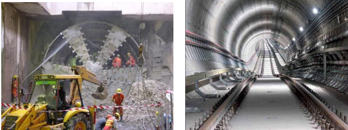
Fig. 7 Some tunneling activities for the MRTA system in Bangkok
