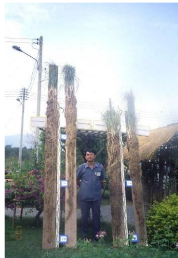
Fig. 12 Challenging situations for slope engineering in Thailand, Construction of reinforced soil slope, vetiver grass utilization and soil blanket in slope protection
