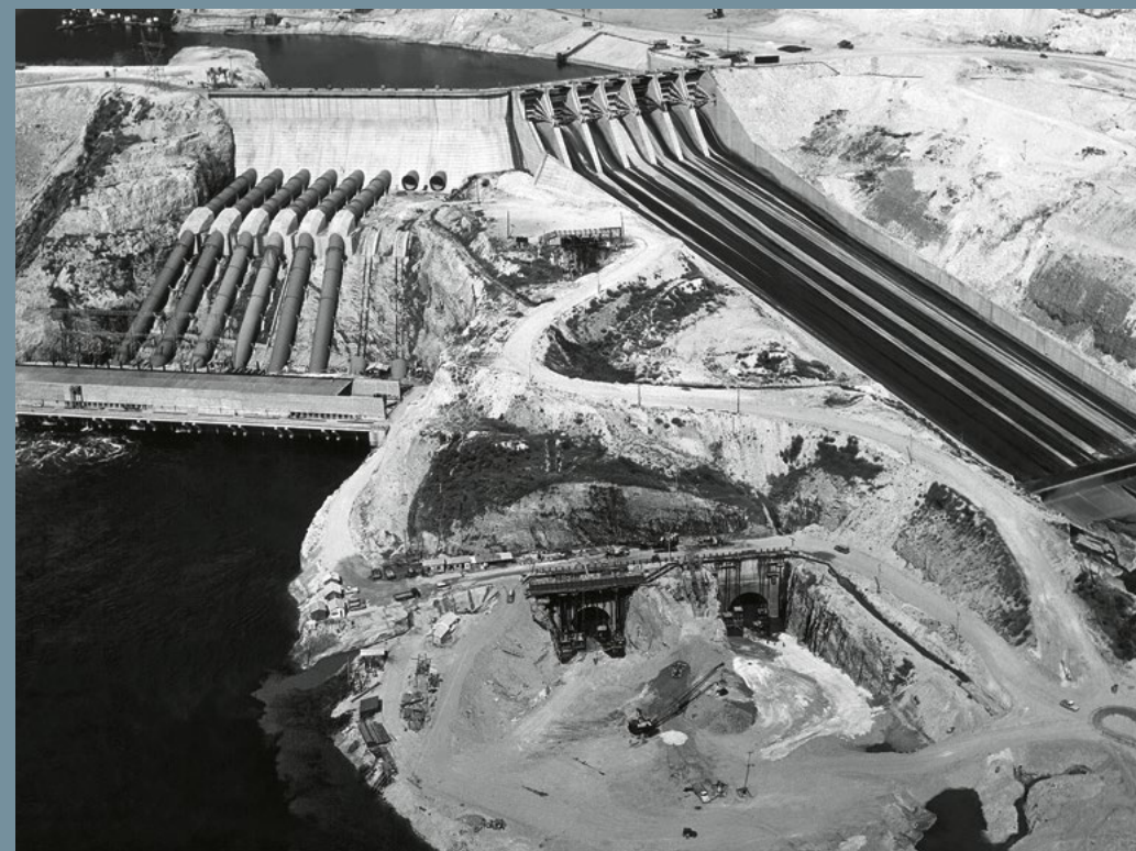
Aerial view of the dam and quarters of the Furnas plant. Furnas CEO John Cotrim (on the right), watching the construction works. Power house tunnel. Penstocks, power house and spillway.
