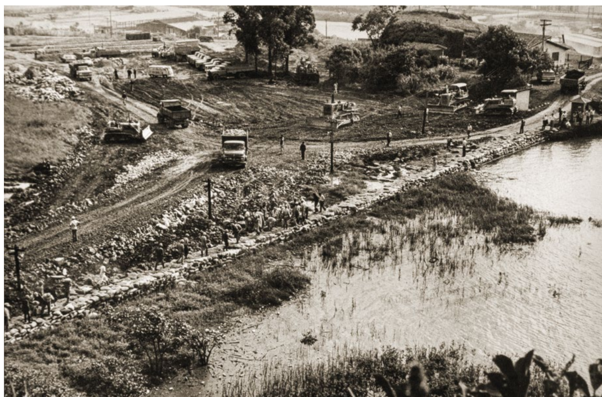
Construction of the Guarapiranga reservoir by Light: in the background, the Pinheiros River downs and the timid Santo Amaro borough, 1907. View of the Guarapiranga dam with the sandbag barrier and earth filling works in the downstream area, January 30, 1976. The measures were Victor's suggestions to keep the reservoir from overtopping.
