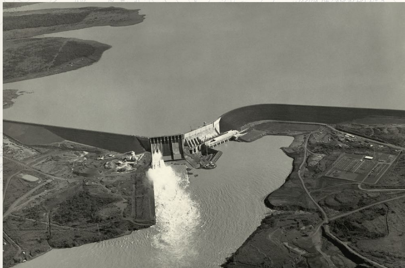
São Simão dam, on the Paranaíba River, at the MG-GO state border, a massive project unveiled in 1978.
