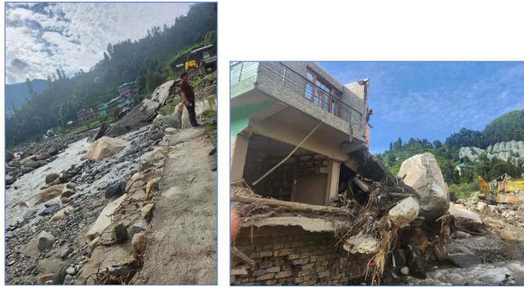
Figure 15. Landslide in Pandav Shila a) Eroded banks b) Flow-Structure interaction caused house collapse
