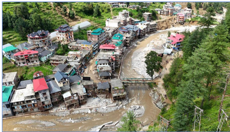
Figure 16. Landslide near Thunag Valley caused river damming and bank erosion
