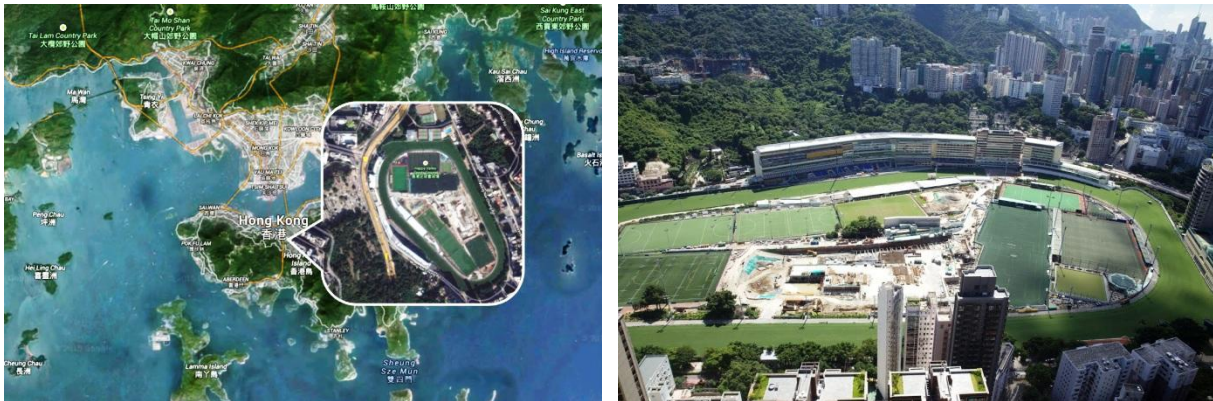
Figure 2. Location of HVUSSS project site; Insert: Project site in Happy Valley Recreation Ground, surrounded by the horse-racing field of the Hong Kong Jockey Club (Images from Google Map)
