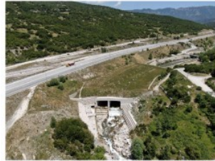
Twin tunnel of Messolonghi River with berms above it stabilizing one landslide to the north (left side) and to the south (right side). Picture taken by drone from downstream of the river.
