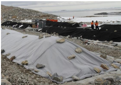
Figure 9. Geotextile covered biopiles in summer
