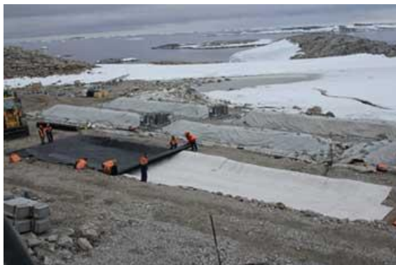
Figure 7. Installing geomembrane over GCL liner
