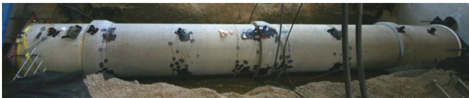
Figure 6. Reinforced concrete pipe prior to burial and testing under surface loads.
