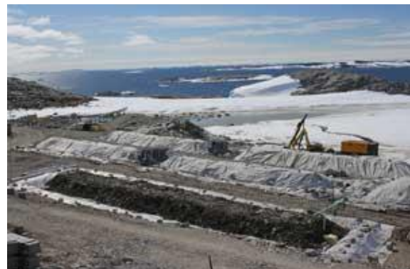
Figure 8. Filling biopile with contaminated soil
