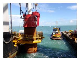
Installation of monopole foundations for the London Array
