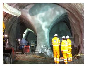
Instrumenting a new SCL tunnels with fibre optics
