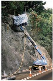
Figure 7. Mobile Platform for Soil Nailing Works
