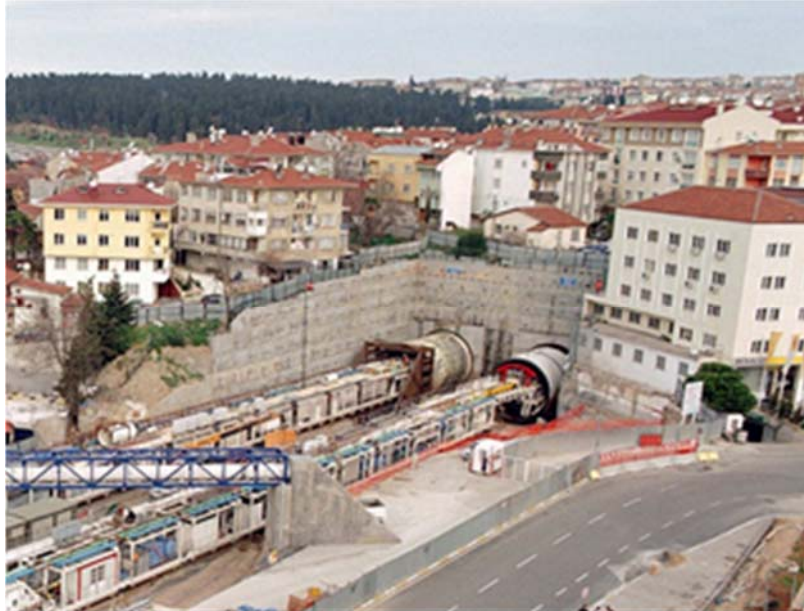
Fig. 5-2 Excavation in an urban area
