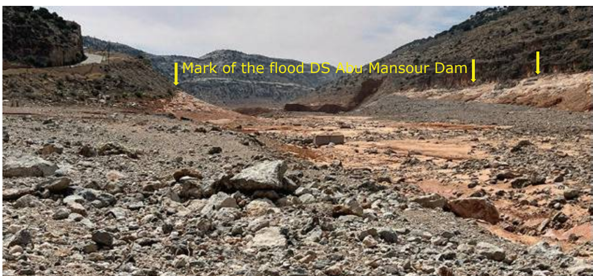
PHOTO 4.5. The view of the downstream of Abu Mansur dam.
