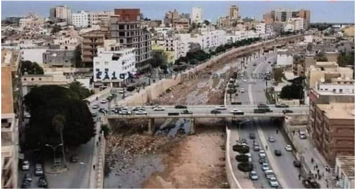
PHOTO 3.1. The Wadi Derna watercourse before the 2023 flood event.
