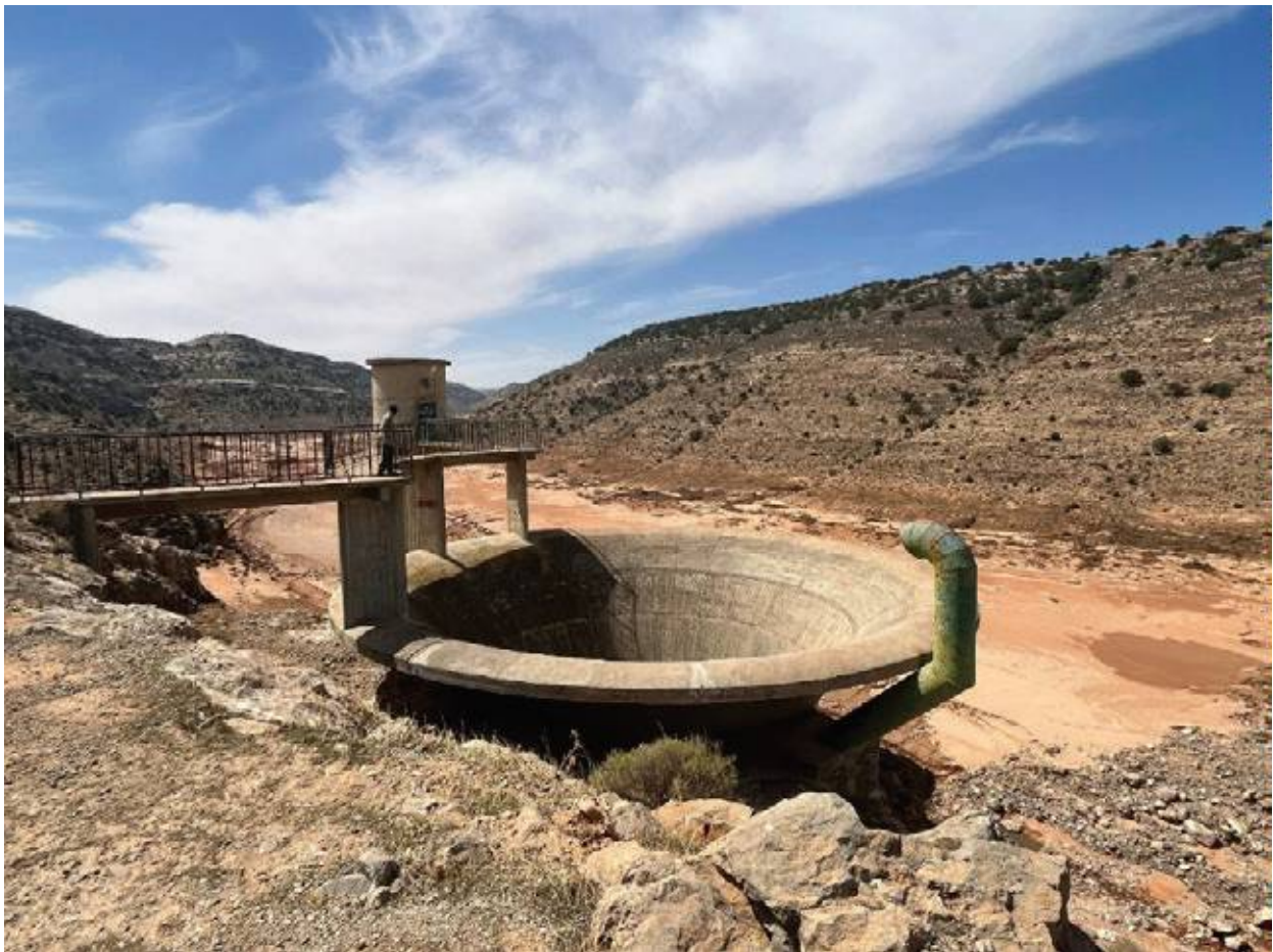
PHOTO 4.7. Morning glory spillway at the Abu Mansour Dam.
