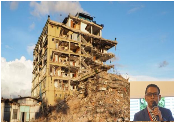
Earthquake in Myanmar, H. Hazarika, March 2025
