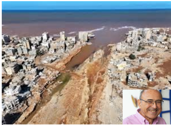
Derna dam, Libya, A. Chraibi, Sept. 2023
