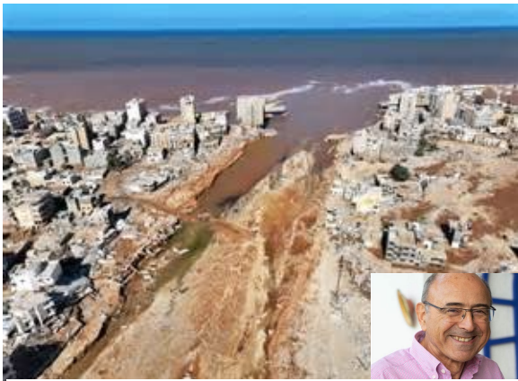
Derna dam, Libya, A. Chaibi, Sept. 2023
