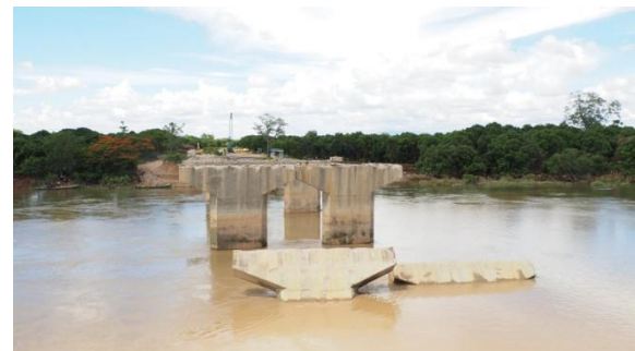
(b)View from the south
