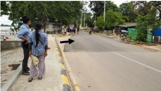
Photo 12: Right-lateral fault dislocation in Sagaing (Left bank of the Ayeyarwady River, near Mandalay)
