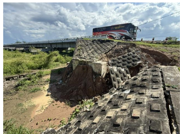
Photo 2: Abutment damage
