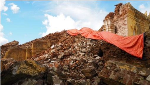
Photo 16: Destroyed Me Nu Brick Monastery in Inwa.
