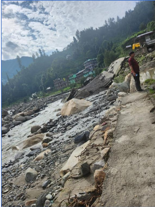
Fig:8 Landslide in Pandav Shila a) Eroded banks b) Flow-Structure interaction caused house collapse
