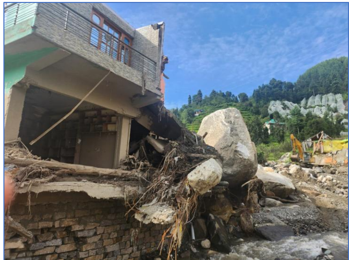
Fig:8 Landslide in Pandav Shila a) Eroded banks b) Flow-Structure interaction caused house collapse
