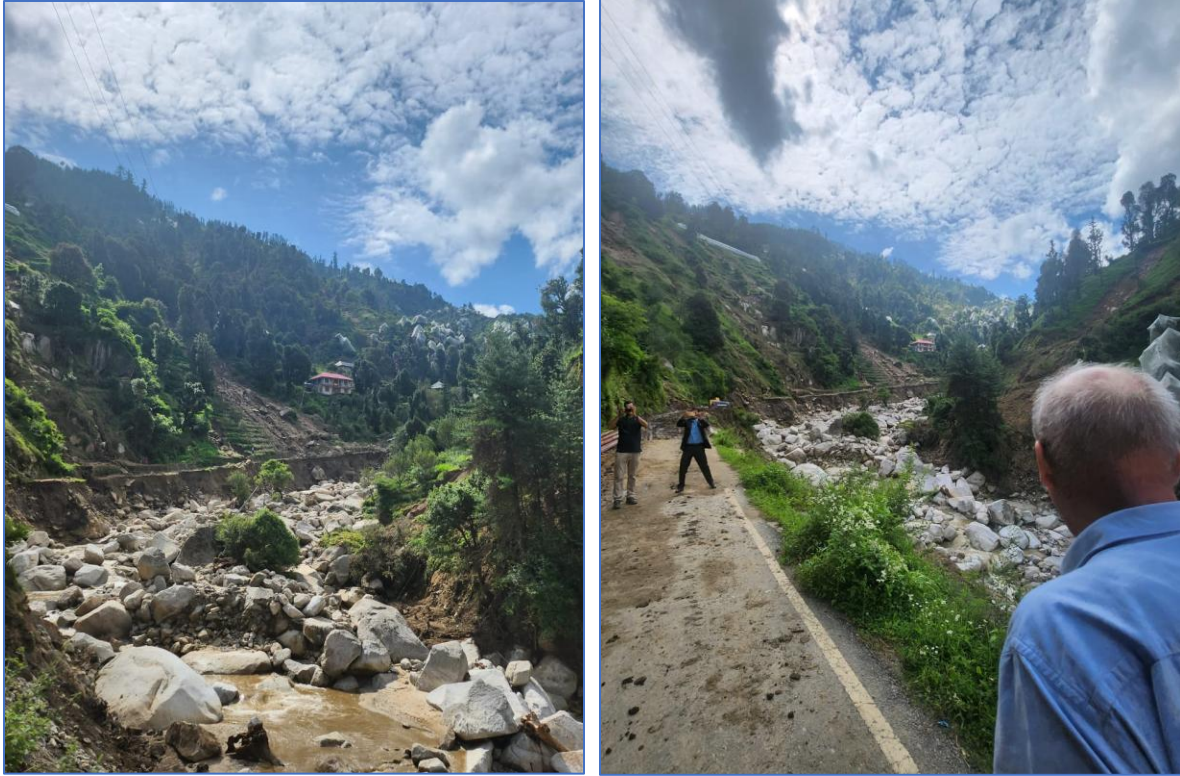
Fig:10 Landslide near location 6 a) Big size boulders present in drainage channels b) Drainage gully is dammed with granular flow
