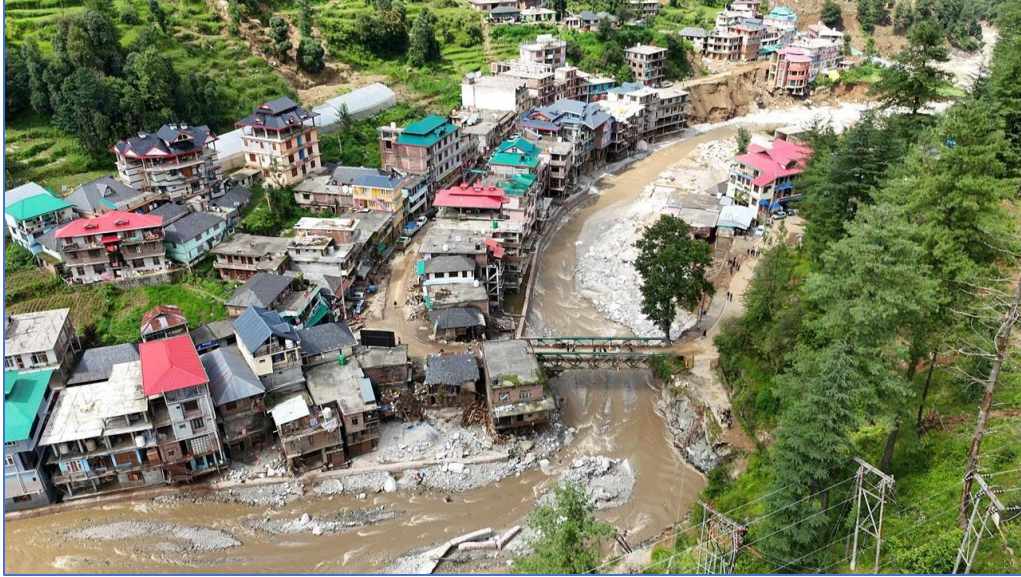
Fig:12 Landslide near Thunag Valley caused river damming and bank erosion
