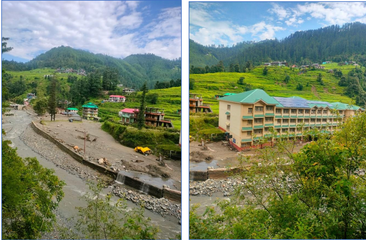
Fig:9 Landslide near Seraj College a) Debris flow damming river channel b) College building submerged with debris/slurry
