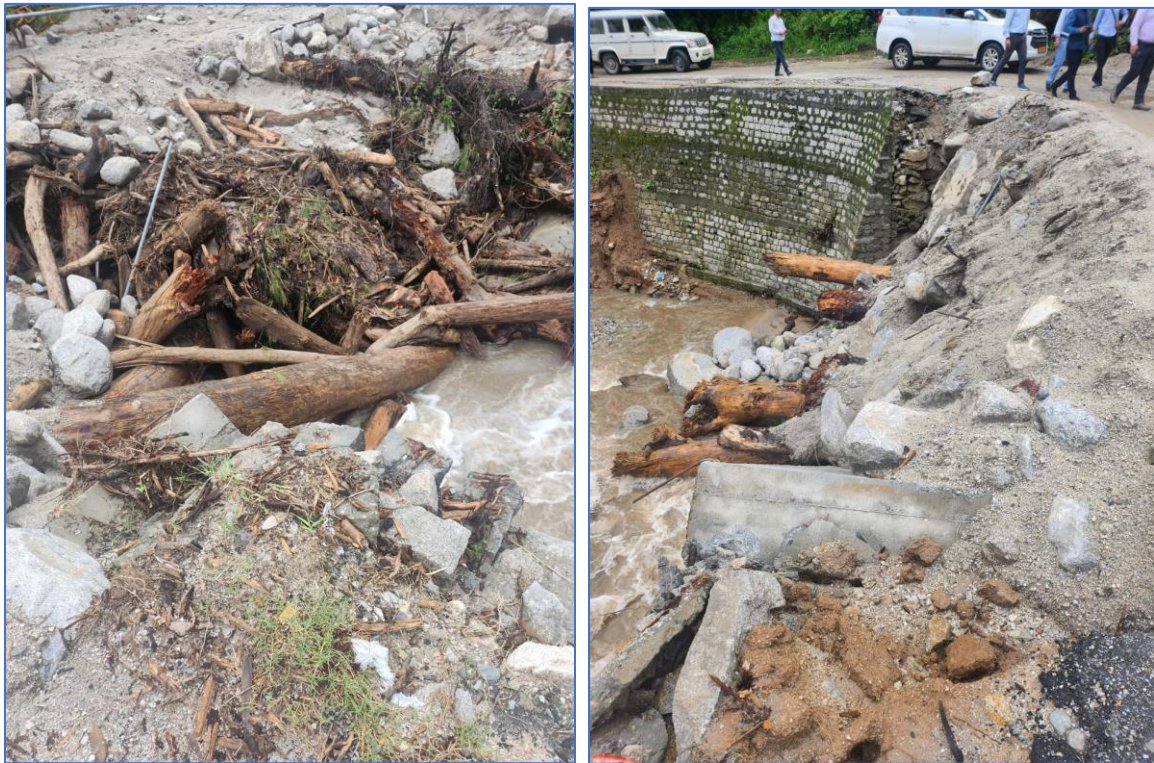
Fig:6 Landslide in Shankar Dera a) uprooting of vegetation b) blockage of culvert due to flowing trunks/roots of vegetation
