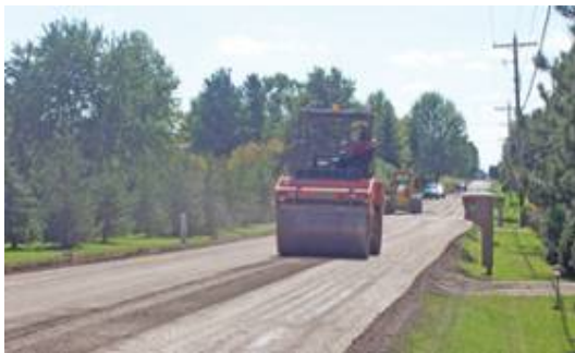
Figure 3. Compaction of FDR base
