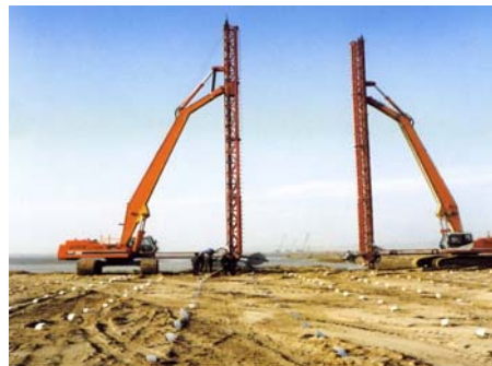
Port Reclamation using Vertical Drains
