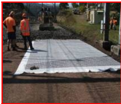
Rail Track improvement using Geosynthetics
