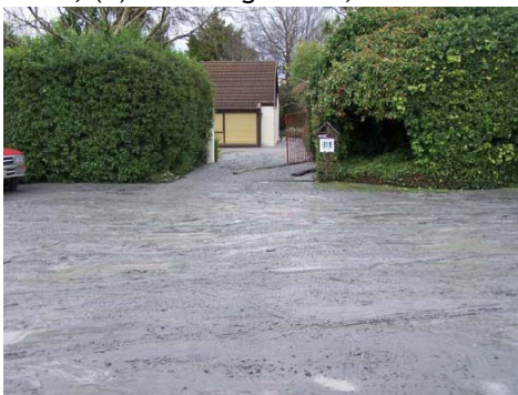
(c) View from the street (before clean up); (d) liquefied silt-sand-water mixture covering a rug inside the house and the ground outside the house (seen through a window from inside the house)
