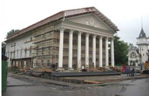
Figure 1. General view of the theatre during reconstruction
