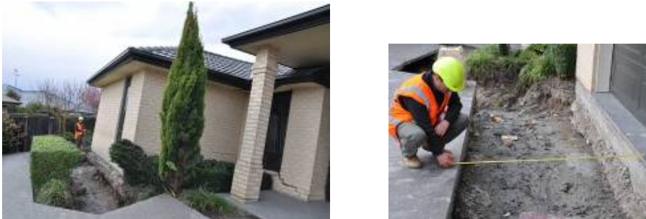
Figure 11. Severe damage to residential houses/properties due to lateral spreading in South Kaiapoi; (a) Excessive tilt and uplift of foundations due to lateral spreading; (b) The width of this crack increased from 1.4m to 1.6m in the period between 11 and 15 September (7-11 days after the mainshock).
