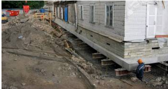
Figure 3. Suspension of the building on Titan piles to provide construction of the rigid disc slab
