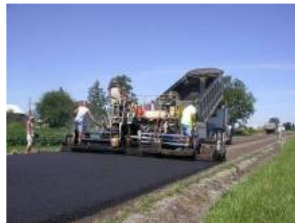
Figure 4. Resurfacing with hot mix asphalt
