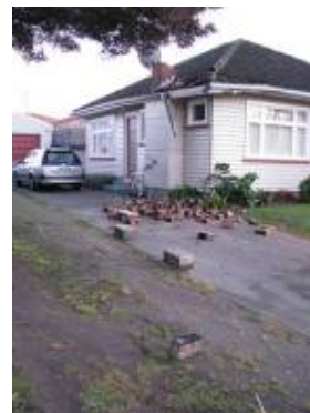
Photo 3: First light: typical chimney debris of a house in adjacent street
