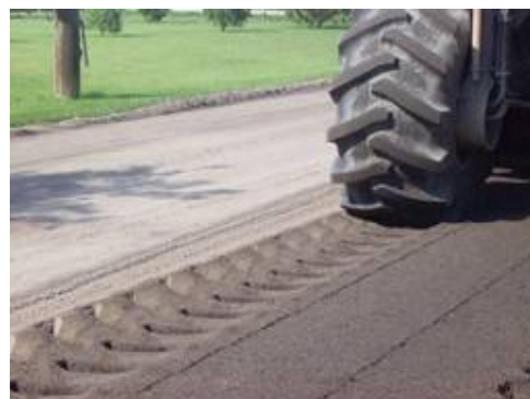
Figure 2. Blending fly ash with pulverized base
