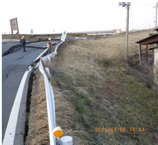
Fig. 33 Distortion of Shida Bridge approach Naruse River, north of Sendai
