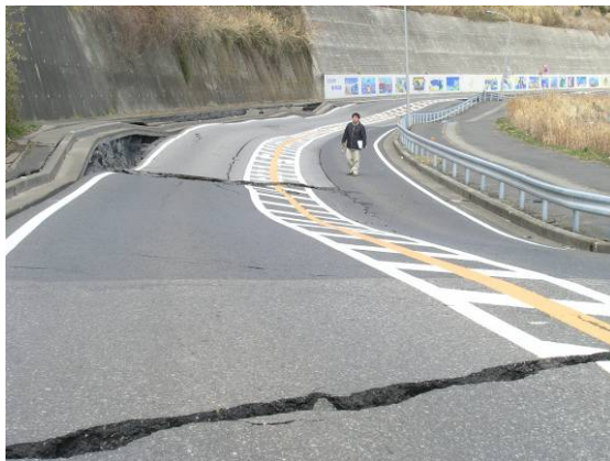
Fig. 21 Distortion of road embankment in Nakaminato of Ibaraki Pref.
