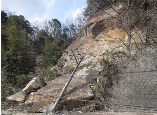
Fig. 31 Rock fall at Ohgo of Ibaraki
