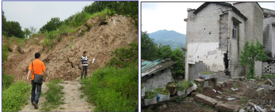
Fig. 17 Failed slope at Three Gorge Dam Reservoir
