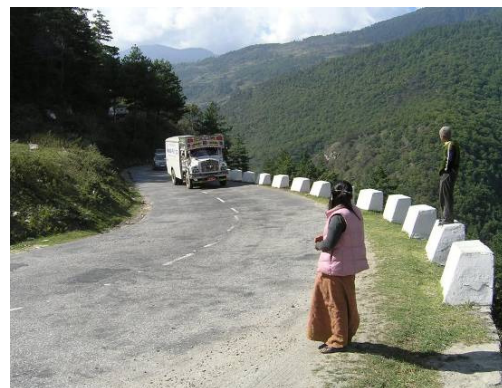
Fig. 3 The highway connecting Thimphu and Phuntsholing.
