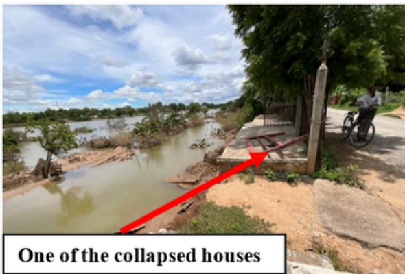
Photo 6: Landslides and collapse of houses
