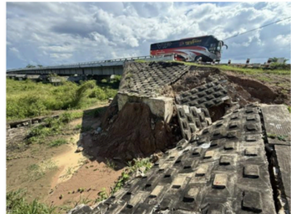
Photo 2: Abutment damage
