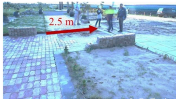
Photo 13: Fault dislocation in a solar power station
