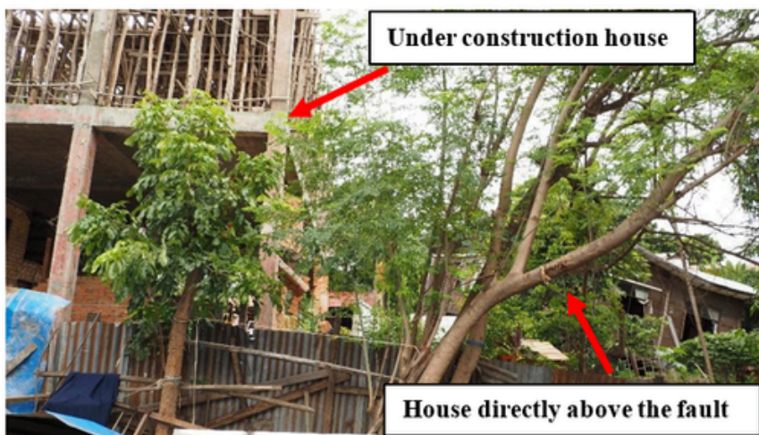
Photo 14: Contrast of damage of two adjacent houses on the opposite side of fault dislocation in Photo 12
