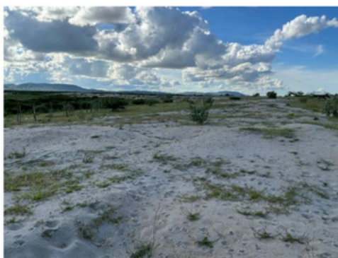
Photo 3: Sand boils at shopping mall site
