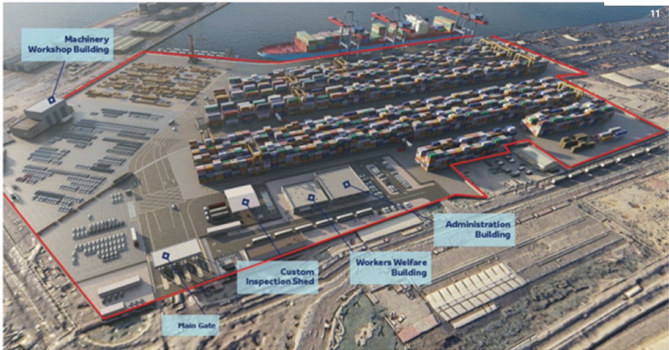
Figure 11 The locations of the main buildings.
