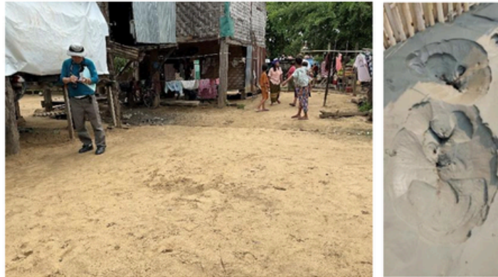
Photo 9: Traces of sand boils in the village
