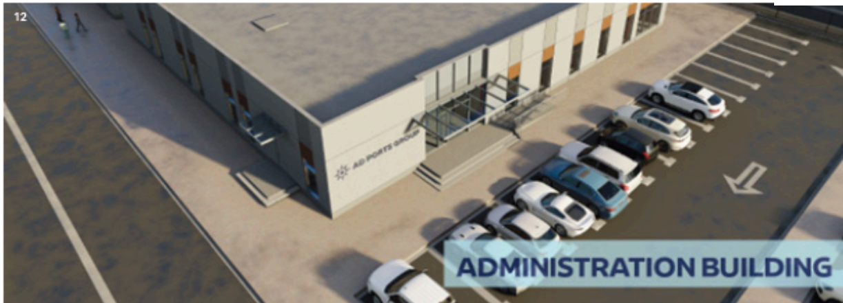
Figure 12 The Administration Building.
