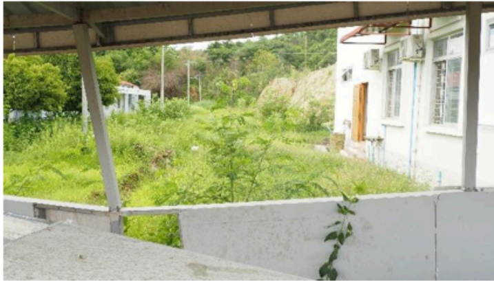
(e) Continuation of fault rupture on the northern side of the site
