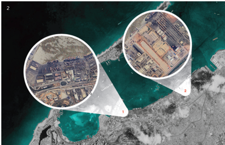
Figure 2 The locations of the Unicargas Terminal (1) and the Temporary Yard (2) within the Port of Angola
