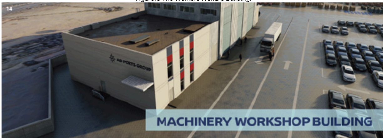
Figure 14 The Machinery Workshop Building.
