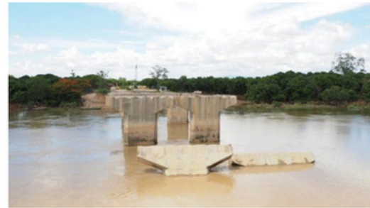
(b) View from the south
