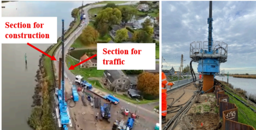
a. Overview of jobsite
