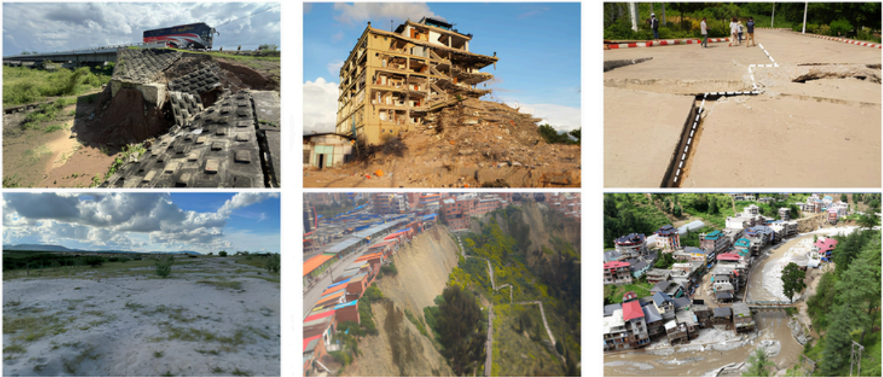
Top: Myanmar 2025 — abutment damage on the Yangon–Mandalay highway; the Sky Villa condominium, Mandalay; fault rupture at the Children’s Specialized Hospital, Naypyidaw. Bottom: sand boils near Naypyidaw; unsaturated-soil slope in La Paz, Bolivia; cascading failures in the Thunga valley, Mandi, India.
