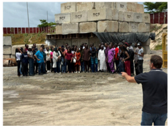
Delegates tour reclamation and foundation works on site.
