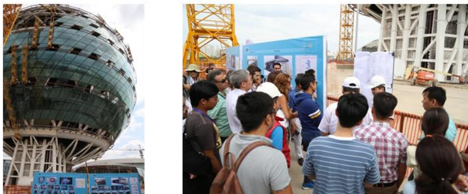
Fig. 7. The EXPO 2017 construction site
