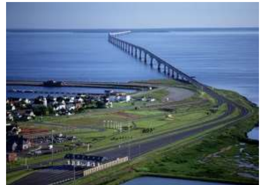
After completion of construction (1998).
