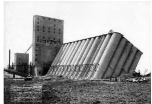
Elevator after failure.
