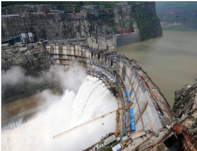
Xiluodu Concrete Gravity Arch Dam, 13860 MW, H = 285.5 m, V = 128x10 8 m 3
