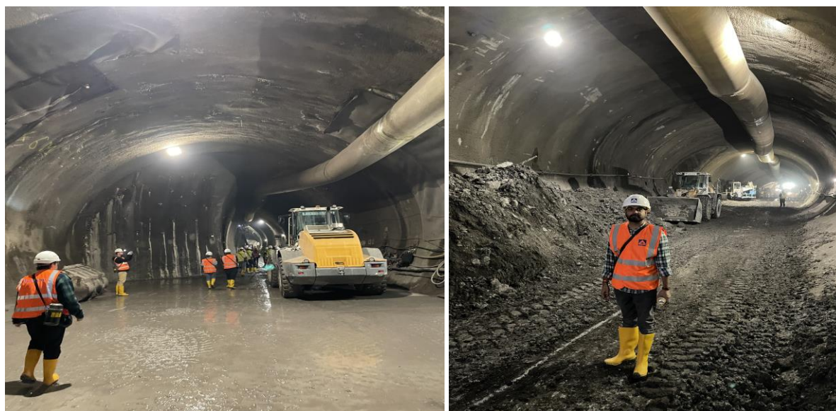
Me at the Site visit of Line D of the Prague Metro – excavation of access tunnels in the direction of Pankrác D Station
