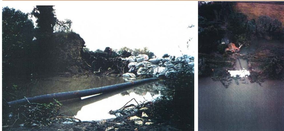
Figure 4.10 Scenario n°2: Breach by concentrated leak erosion in a hole along a crossing structure.
