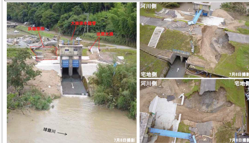
Figure 3.33 Example of overtopping from the presentation 'Picture-Card Show Project' in JGS-JCES', contribution by K. Maeda, M. Ishihara and H. Mori, using materials from the Ministry of Land, Infrastructure, Transport and Tourism in Japan.
