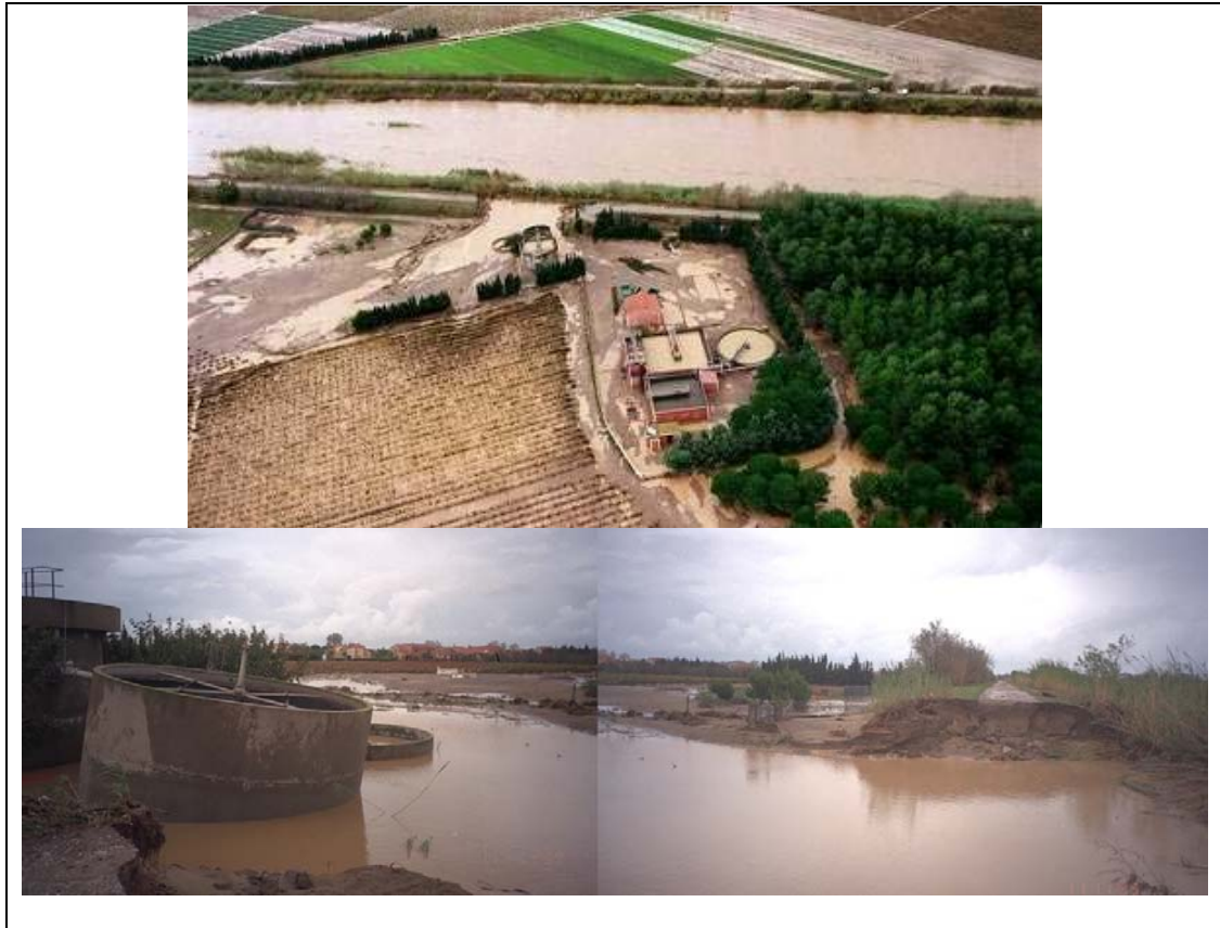
Figure 3.49 Breach in 1999 at St-Laurent-de-la-Salanque.
