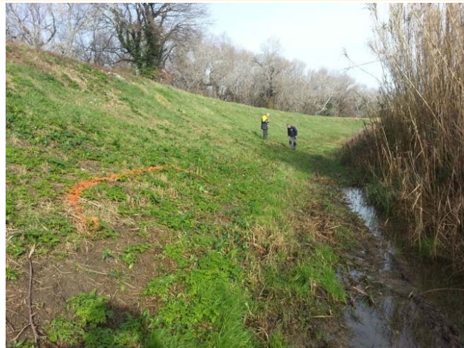
Figure 4.12 Scenario n°4: Breach by concentrated leak erosion in a crossing crack along a former transition insufficiently treated.
