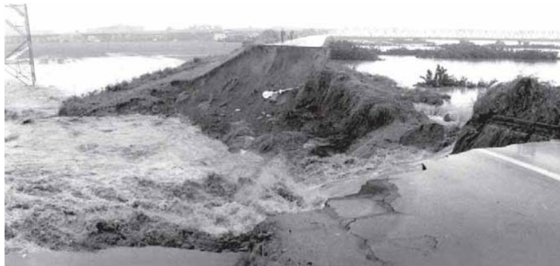
Just after breach
