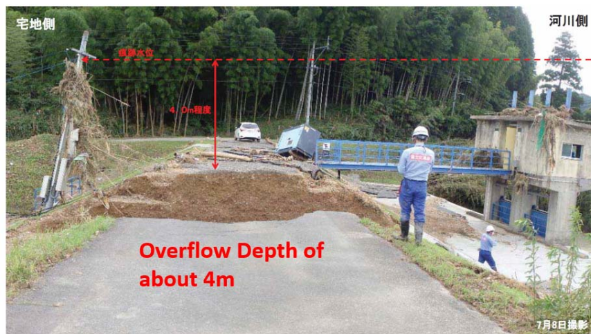
Figure 3.32 Picture of overtopping from the presentation 'Picture-Card Show Project' in JGS-JCES', contribution by K. Maeda, M. Ishihara and H. Mori, using materials from the Ministry of Land, Infrastructure, Transport and Tourism in Japan.
