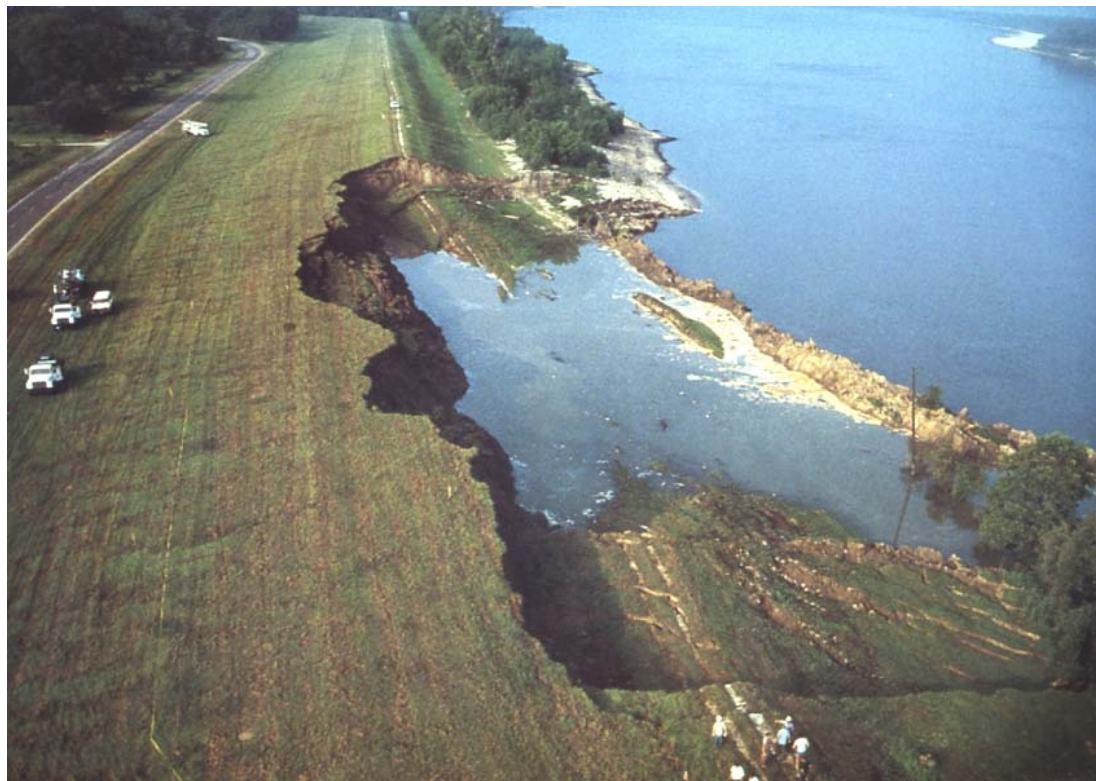
Figure 3.64 Photo: This 210 m section of levee slid into the east side of the Mississippi River on August 23, 1983 at Darrow, in Ascension Parish, Louisiana. The slide occurred shortly after a high-water stage had receded, suggesting that toe undercutting and rapid drawdown likely contributed to the failure.
