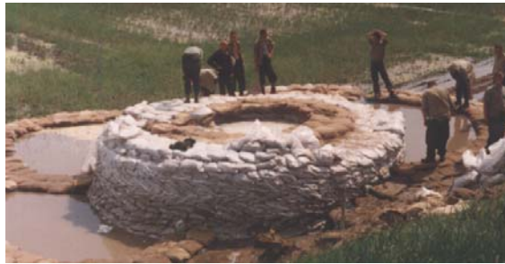
Figure 3.39 Counterpressure basin for related cassettes (left) and location of sand cassettes (right).
