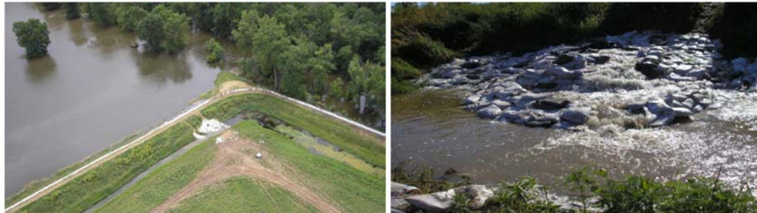
Figure 3.9 Seepage occurring at the toe of the levee prior to breach (taken around 0800 hr, 23 June 2008) (left), and Sand bag effort prior to breach (taken around noon on 26 June 2008) (right).
