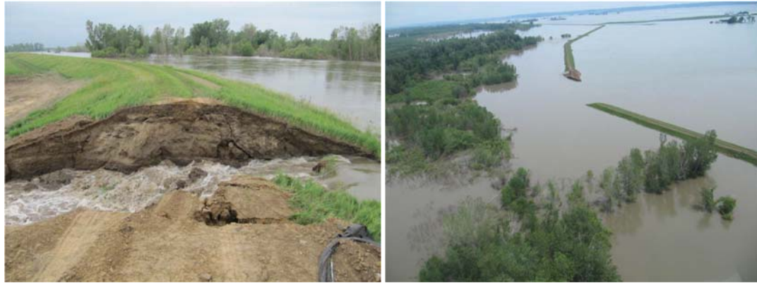
Figure 3.15 The initial breach of the levee L-575 (left), and the levee breach after complete interior flooding (right).
