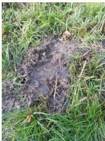
Figure 4.12 Scenario n°4: Breach by concentrated leak erosion in a crossing crack along a former transition insufficiently treated.
