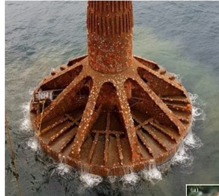
Dogger Bank Met Mast Removal 2017 after 4 years operation (photos: SPT)
