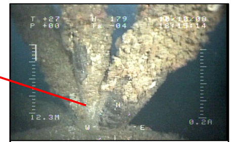
Cracked and damaged joint
