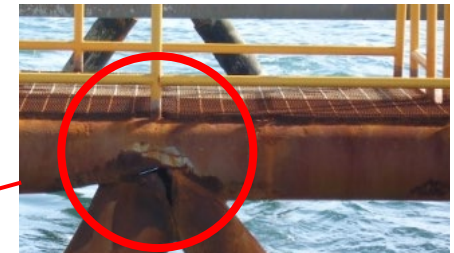
Joint failure and separated members
