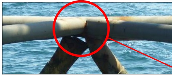
Joint failure and separated members
