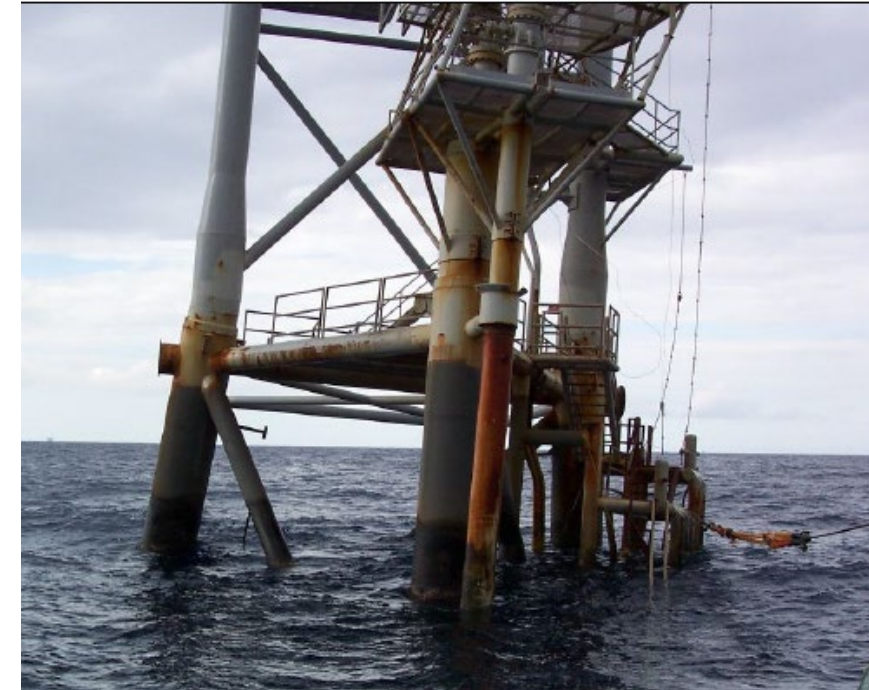
Platform leaning beyond repair in East Cameron area
