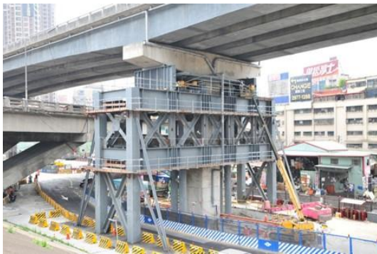
Figure 10 Underpinning P64 in progress
