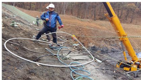
(b) Packing and pressurized grouting
