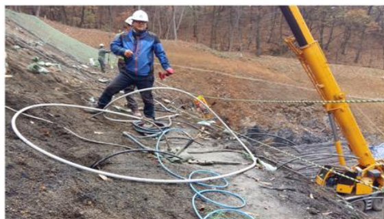
(b) Packing and pressurized grouting
