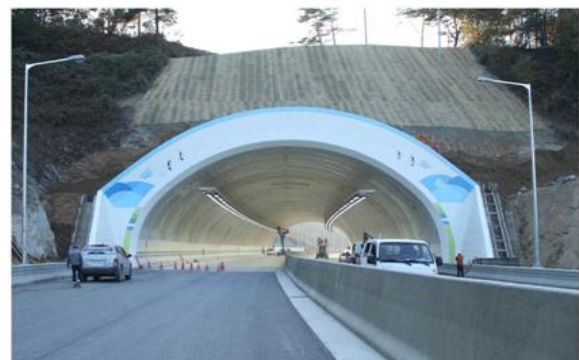
(b) Tunnel completion with concrete lining
