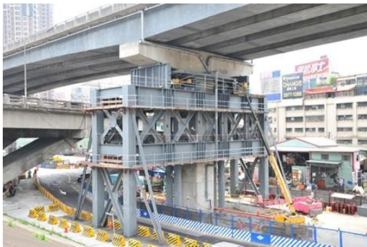
Figure 10 Underpinning P64 in progress
