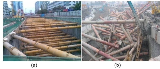
Figure 14. Retaining system of deep excavation and its failure at Xianghu Station of Hangzhou Metro Line 1 (a) Excavation retaining system (b) Failure scene of the retaining system.
