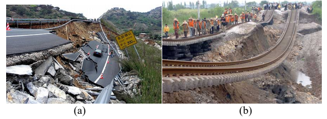
Figure 36. Photo of the embankment failure in (a) Luochang highway and (b) Railway subgrade.
