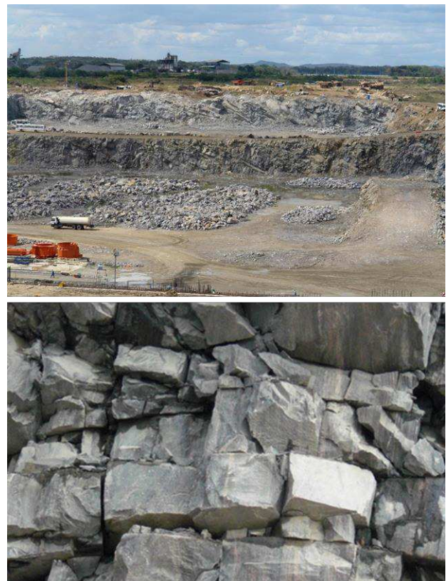
Figure 7. Excavation in the Tocoma discharge channel, estado Bolívar, Venezuela. Igneous rocks mass with the presence of sub-horizontal joint patterns, limiting sub-vertical joint planes.
