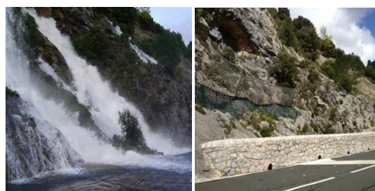
Figure 8 Situation of PK 158,140 MI produced by heavy rains and situation of PK 158,140 MI with the finished stonework (national road side)
