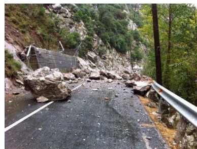
Figure 3. Safety compromised due to stone falling in the road N-621 after intense rains.
