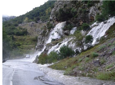
Figure 1. Situation of PK 158,140 MI produced by heavy rains on rocky slope (upstream) without acting.
